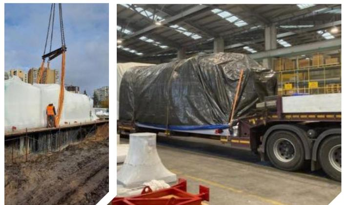
KGE Baltic were invited by their reliable customer to transport a heavy cold module unit with dimensions of 15.6 x 2.7 x 3.4m and a weight of 43tn.
