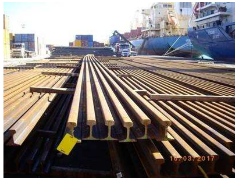
Discharging and Delivery of Rails (L:36m)
