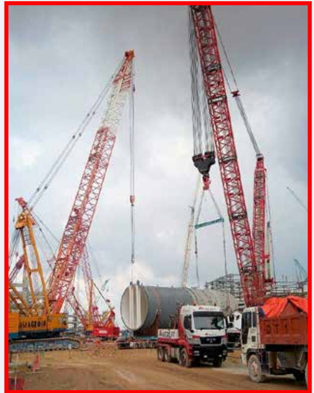
Cargo: Dilution Steam Drum Dimension: L24.30 m x W6.42 m x H6.72 m Weight: 93.86 tons
