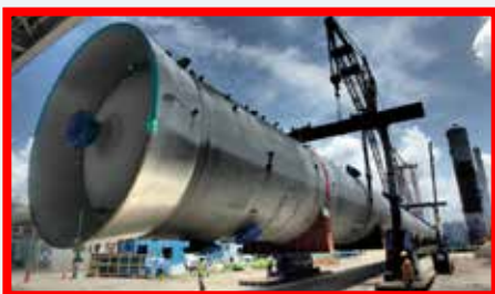
Cargo: Propylene Splitter Dimension: L94.05 m x W5.78 m x H5.08 m Weight: 580 tons Scope: Lifting
