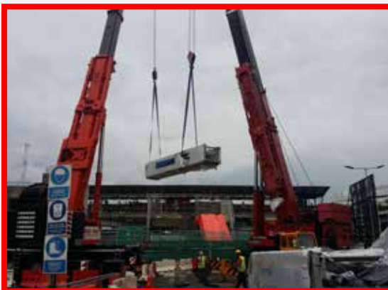
Cargo: Escalator Trusses Various dimensions and weights Scope: Lifting and installation
